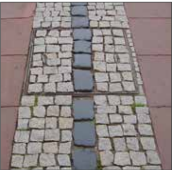
Image 2 - Stone mosaic with a permeable fill between the stones.
