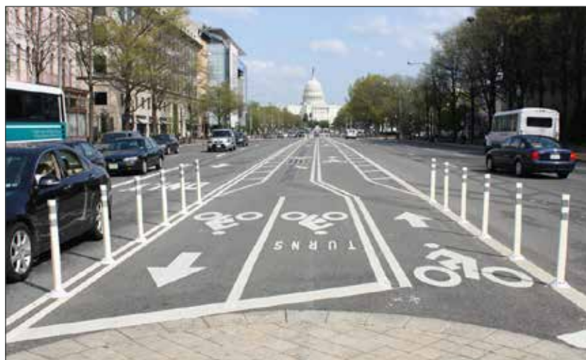
Image 6 - Separated bike lane at intersection with individual turning lanes.
