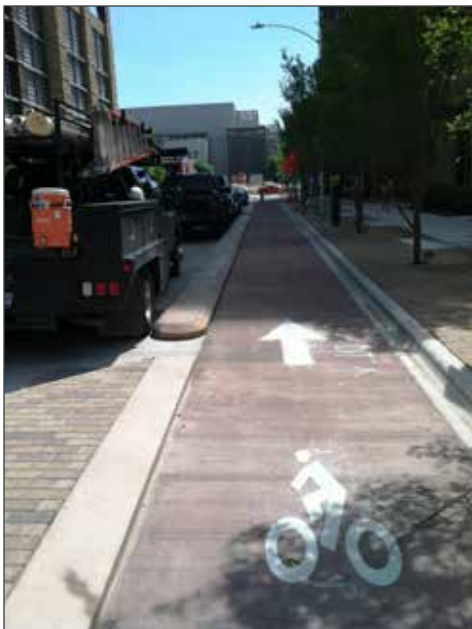
Image 1 - Cycle track separated with concrete and paving.
