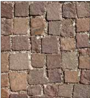
Image 3 - Bricks with sand support a permeable material system.
