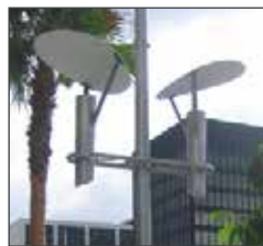
Image 10 - Contemporary fully shielded light fixture bracket mounted at 14' height on a 20' pole - a good method for integrating pedestrian scale lighting with required roadway lighting.
