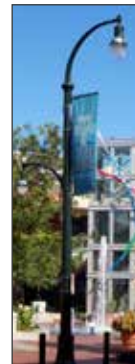
Image 7 - Lamp that uses one fixture at 12 feet tall and an- other fixture at 20 feet tall for vehic- ular traffic.
