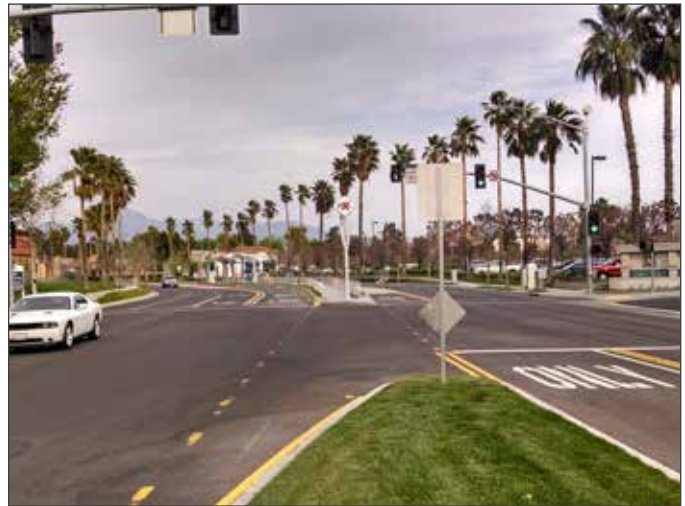
Image 4 - Integrated BRT line on a two-way street.
